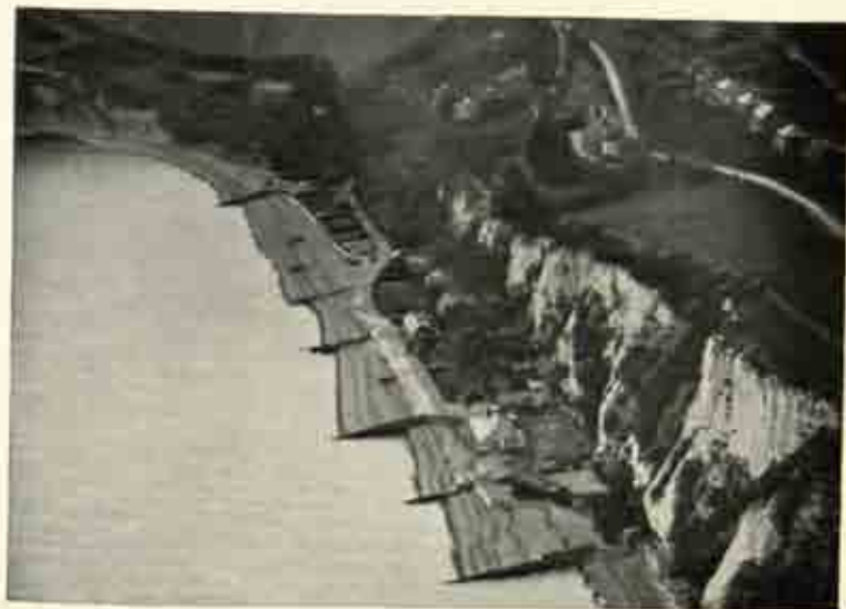
(B) Beach drift impeded by groynes, St. Margaret's Bay, Isle of Wight
